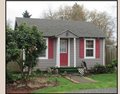
This Minimal Traditional-style house is a one-story, wood-framed box with gable roof and exposed rafters. You will notice the wide shingle siding and one-over-one horizontal, double-hung windows with false shutters. The small projecting gable porch with boxed posts are typical elements of a Minimal Traditional-style house.
