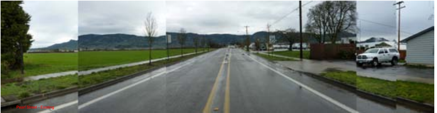
Pearl Street - Existing
