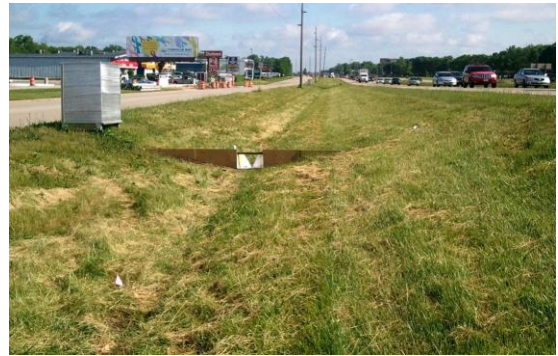
Grassed swale along a divided highway Source: U.S. Geological Survey
