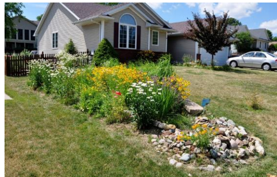
Rain garden on a residential property Source: Stormwater Report, Water Environment Federation
