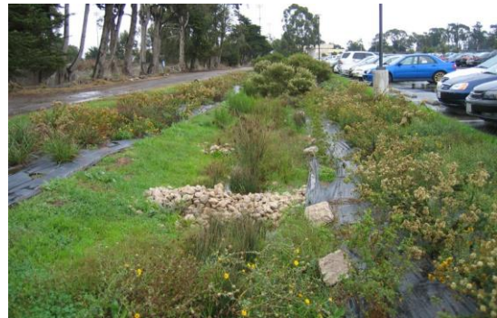
The use of vegetated swale along a surface parking lot Source: University of California, Santa Barbara
