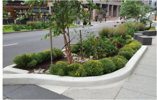
Rain garden as part of an urban green infrastructure Source: U.S. Environmental Protection Agency
