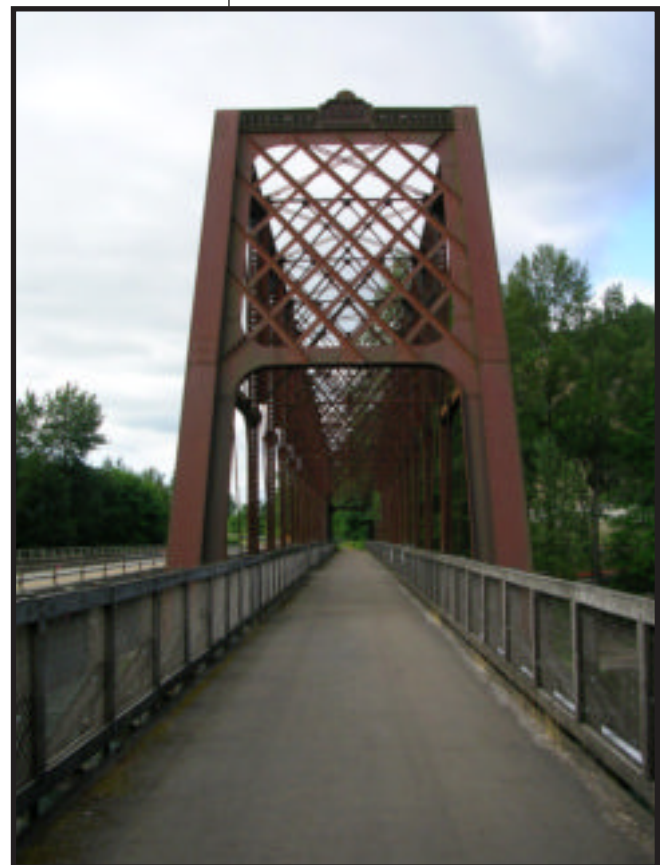
The path will cross the McKenzie River on the existing bicycle/pedestrian bridge near Armitage Park.
